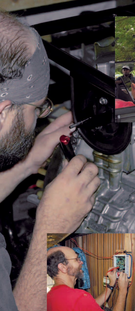
Power players. Andrew Koens (left) works on the team's diesel generators—multiple times over. Brian Chapaitis (inset) tunes translation advisor Beth Fuller's solar electric system.
